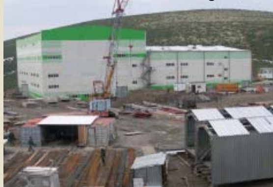
Construction of main building
